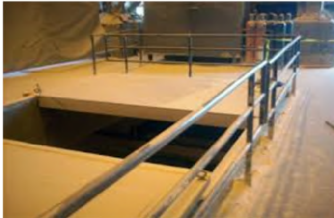
Guardrails around Floor Penetration
